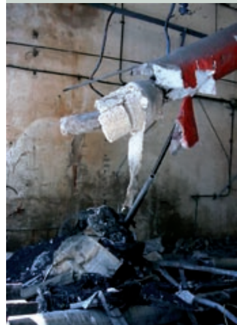
Broken and exposed asbestos piping
