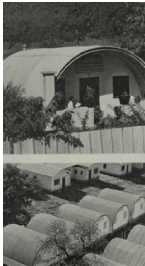
Asbestos cement housing in India
